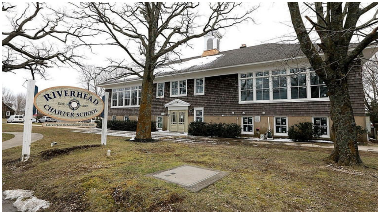
Riverhead Charter Middle School grades 7-8; renovated in 2018.
